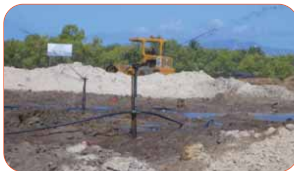
Figure 5 - Moistening of contaminated soil stockpiles
