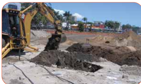
Figure 6 - Piles of hydrocarbon contaminated soil being aerated
