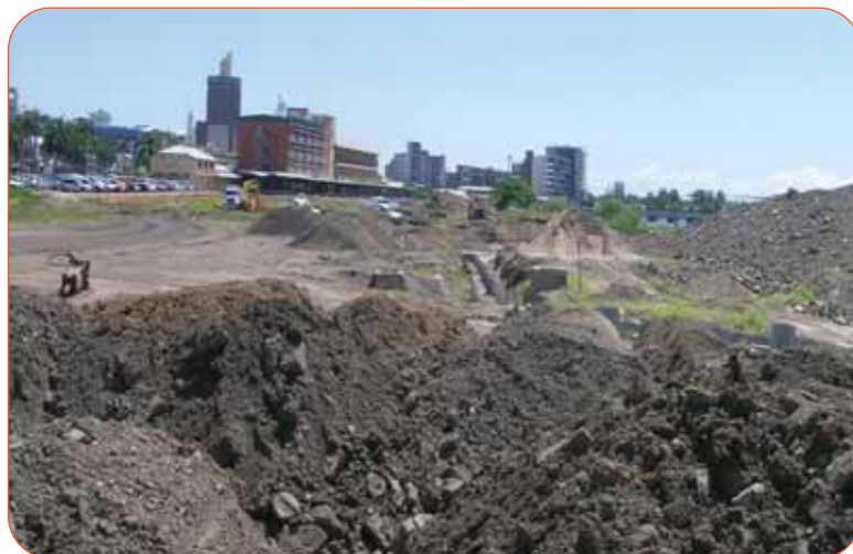
Figure 4 - Contaminated soil that has been piled up ready for ViroSoil™ Technology to be applied
